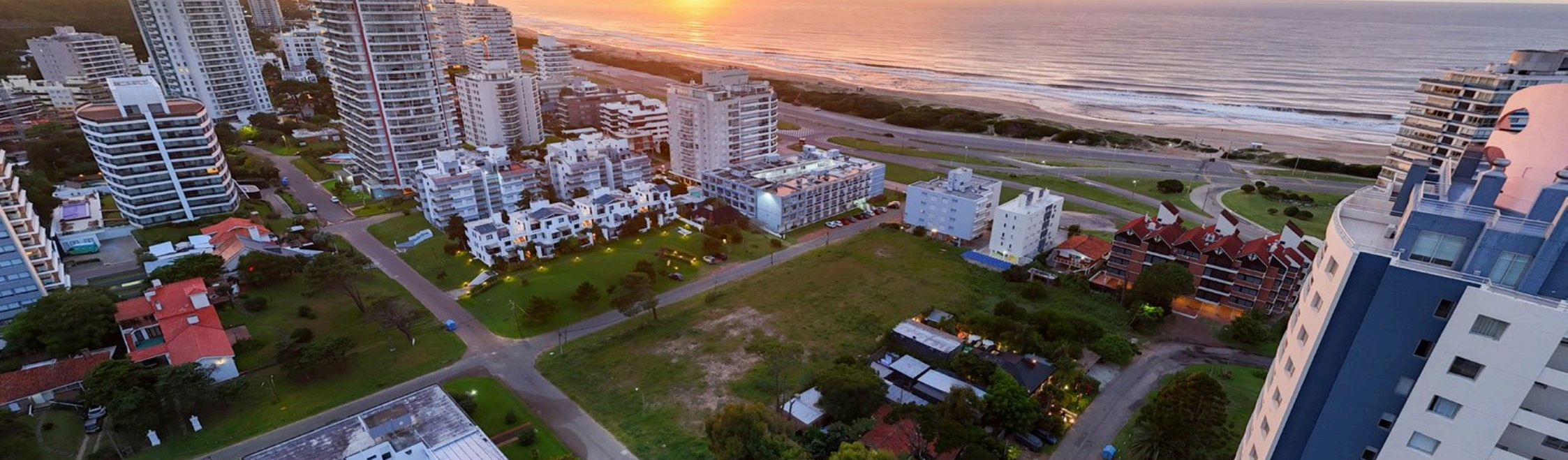
Aerial view of the site at Parada 5. Playa Brava beyond.
